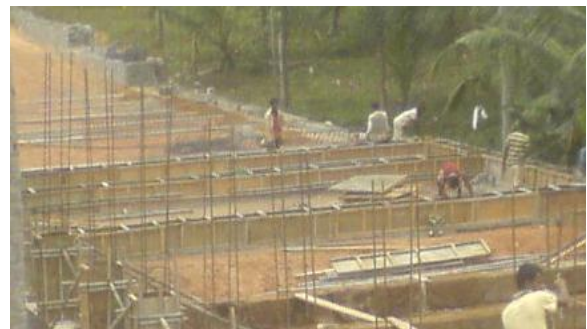
Figure 08: Construction of Connecting Beam at Retaining Wall - Type 3
