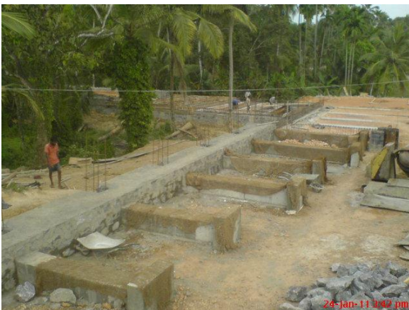
Figure 06: Construction of Anchor Blocks
