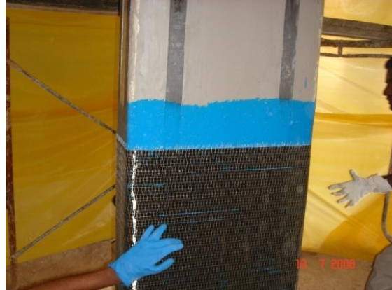
Figure 4: Application of CFRP Sheets
