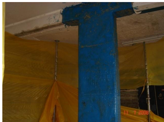
Figure 5: Finished Column before applying plaster
