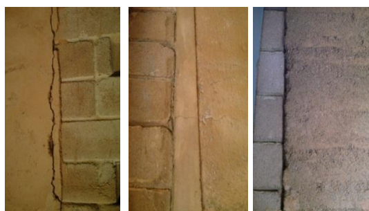
Fig 1: Separation cracks at wall junctions
