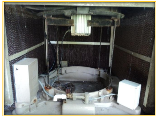
Figure 1: The Pump and the fan within an evaporative cooling unit
