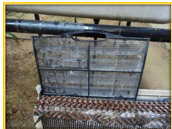
Figure 3: Air filter of an evaporative cooling unit
