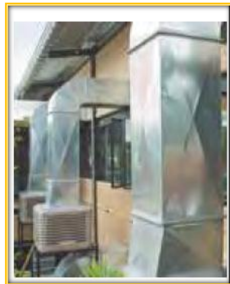
Figure 2: Evaporative cooler are running under non-air tighten condition (Opened windows)
