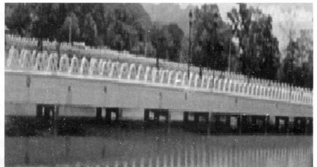
Figure 6: A bridge of 110 m of length and 3.0 m of width constructed at a mere cost of Rs 7.5 million
