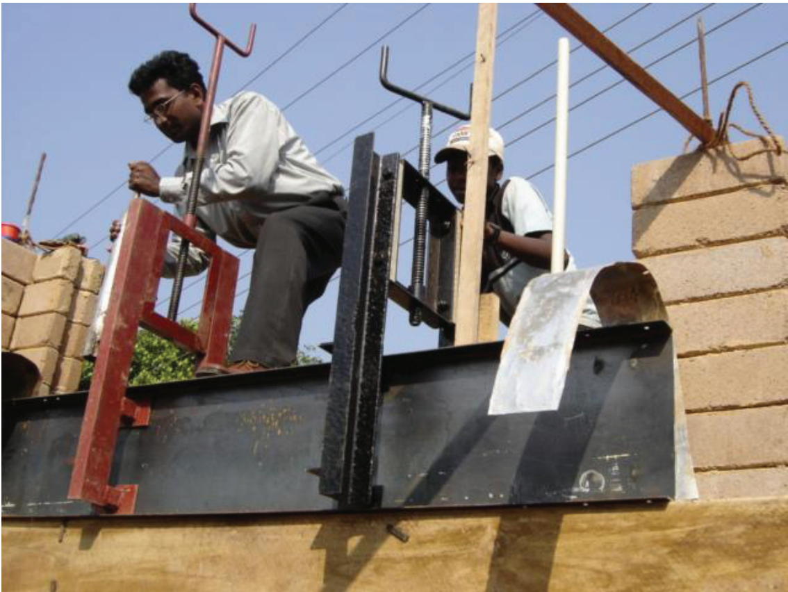
Figure 4: Rammed earth construction
