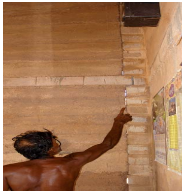
Figure 3 Cracks identified at the wall column junction
