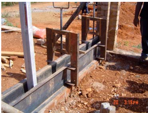
Figure 1 Slip form mould
