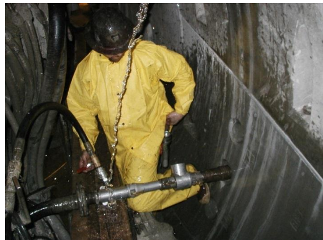
Figure 4: Cellular concrete pumped in the annular gap of a tunnel
