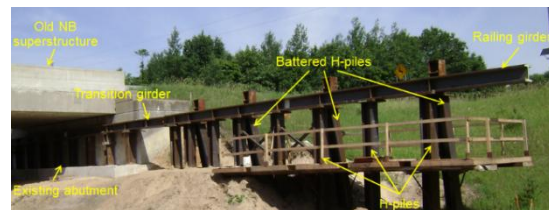
(a) Temporary substructure for US-131 NB
