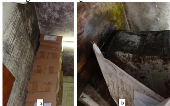
Figure 5: Severe mould growth (a) ICU store room S2 at second floor (b) A duct in S5 at second floor
