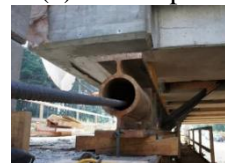
(c) Sliding girder being pulled
