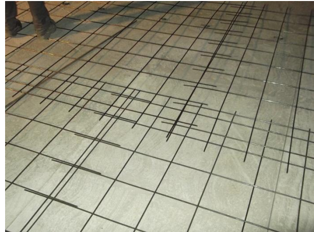
Figure 2: Reinforcement net on a pre-stressed concrete slab panel before prior to screed concreting
