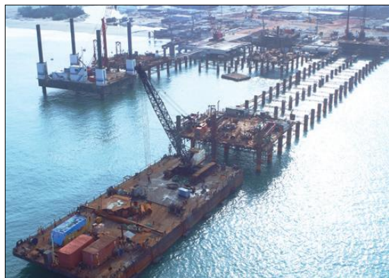
Figure 5: Shiplift under construction
