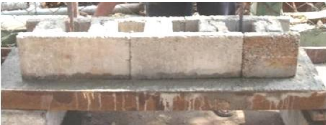
Fig. 4 Photo of wall construction showing interlocking of the blocks
