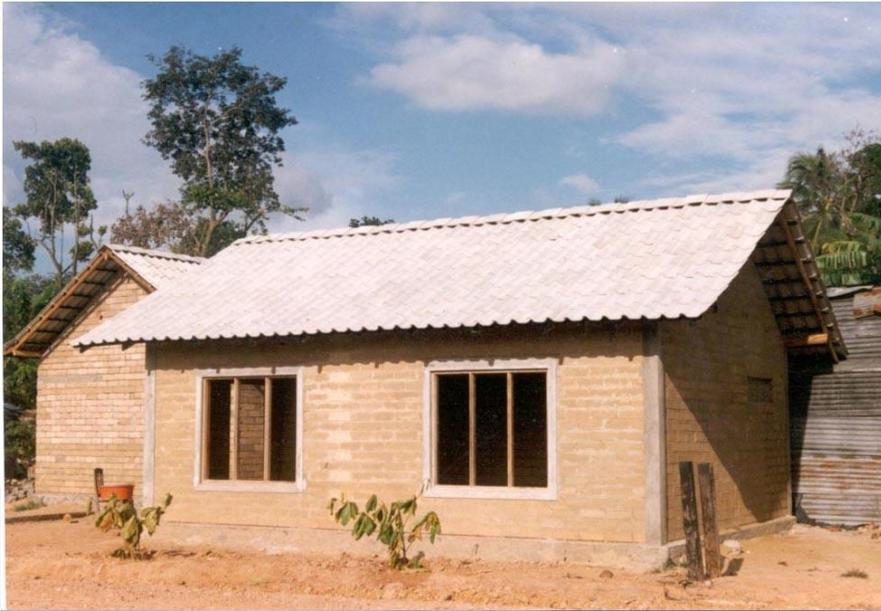
**Figure 1: A house constructed with stabilized soil blocks and MCR tiles**
