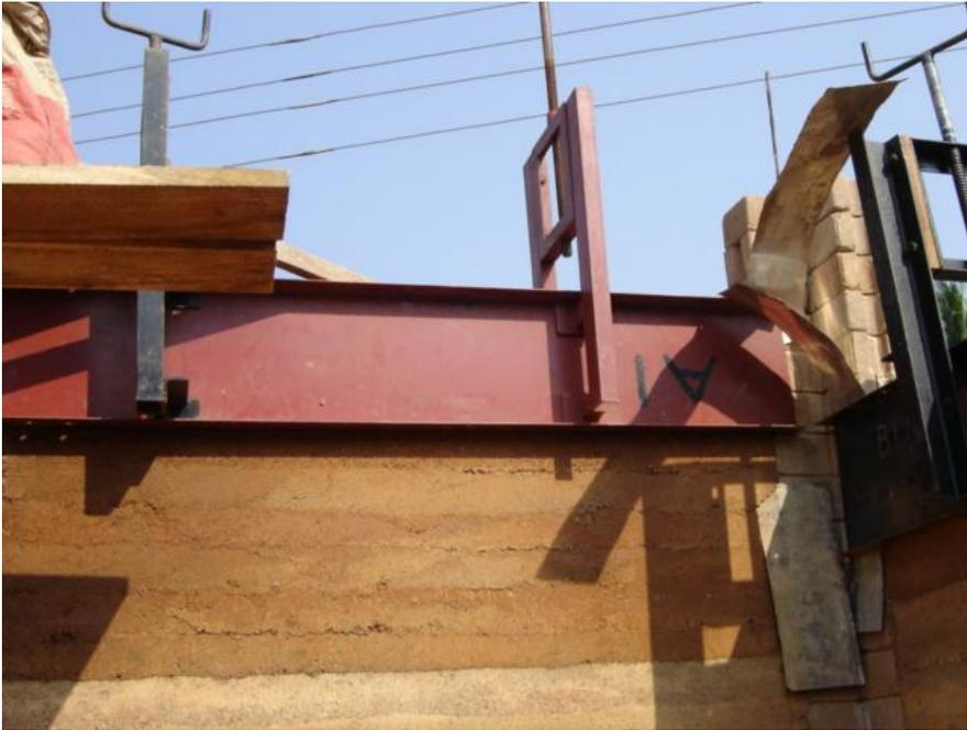
**Figure 2: Rammed earth construction (A photograph taken at Center for Housing Planning and Building, Sri Lanka)**
