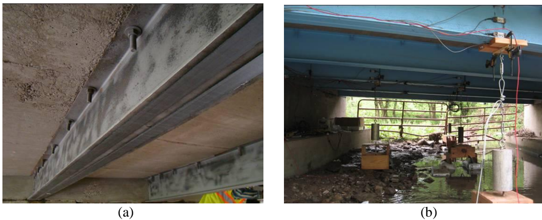
Figure 10: (a) Bridge girder with post-installed shear studs and ultra high modulus CFRP laminates; (b) Instrumentation for field tests
