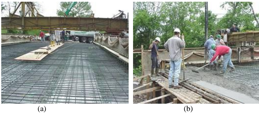
Figure 2: (a) CFRP reinforcements as longitudinal and transverse reinforcement in both the top and bottom mats; (b) concrete placement
