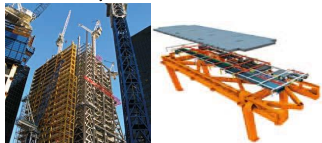
Figure 3: North core and Service integrated bench at The Leadenhall Building (Source: Davies 2013)
