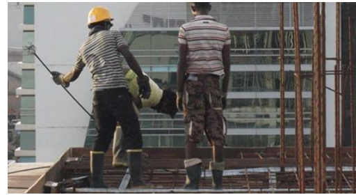
Figure 08 Insert tendons into ducts
