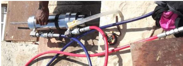
Figure 16: Stressing in progress
