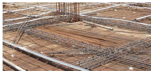
Figure 11: Arrangement of additional reinforcements at the opening
