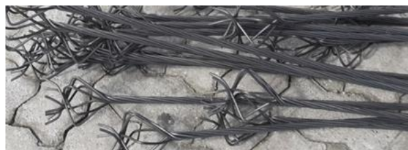
Figure 02: Preparation of dead end anchorage
