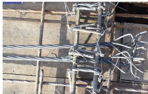
Figure 10 Fixing of bursting reinforcements
