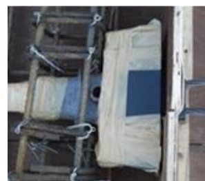
Figure 03: Fixing of pocket formers
