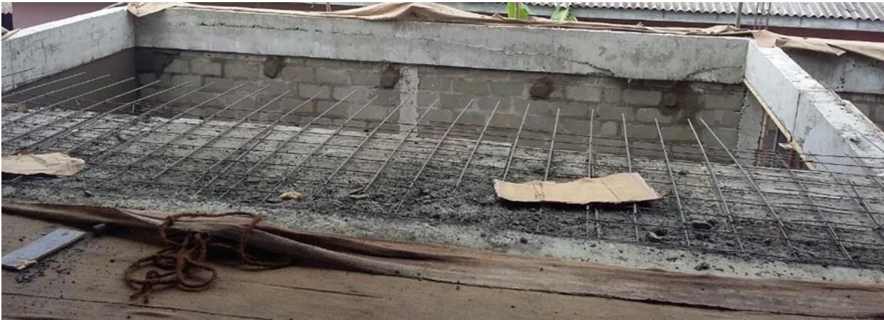
Fig. 07: Slab system with reinforcement
