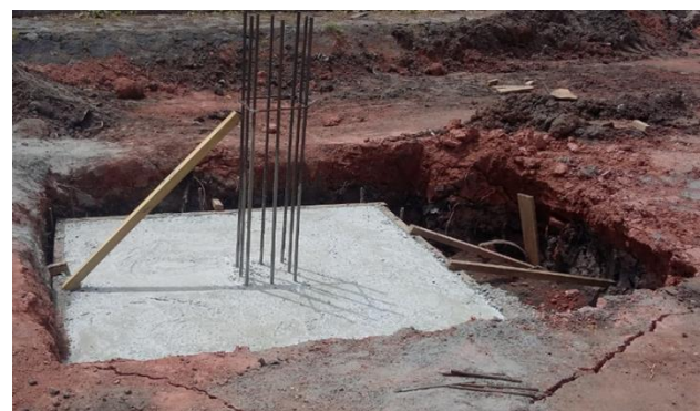
Fig. 02: A pad foundation and the laterite earth compacted filling
