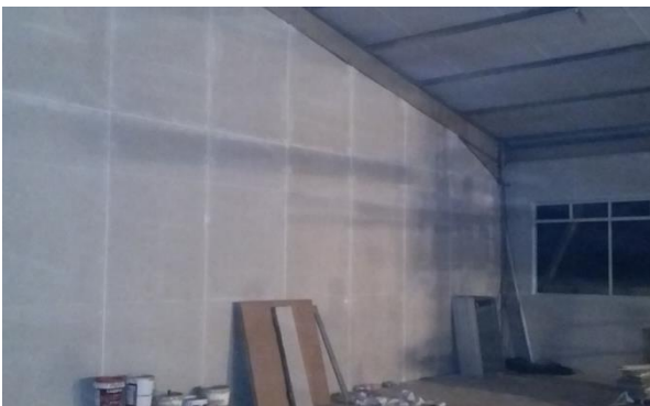
Fig. 05: Completed wall with flexi board mounted compressed straw panels
