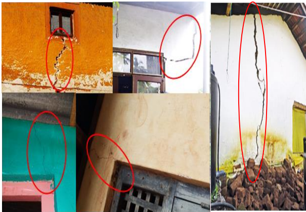
Fig 2: Observed failures of masonry structures - visual observation survey- South East Sri Lanka
