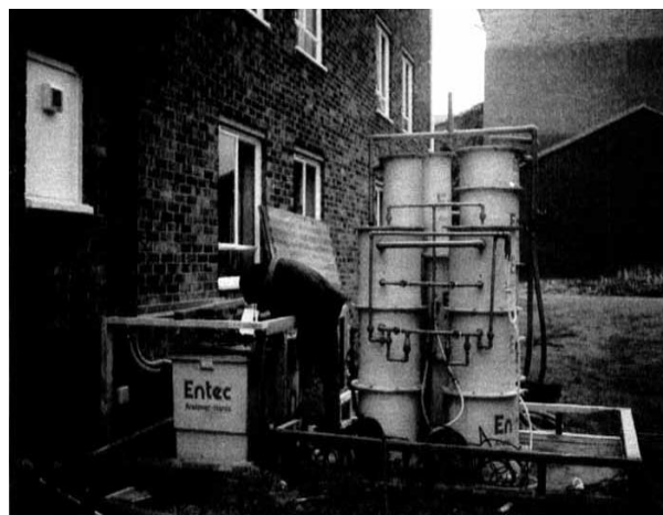
Fig 1: Greywater reclamation Plant construction in Loughborough, source: [5]
