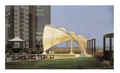
**Fig.12:** This fabric membrane structure at the Hyatt Regency in Osaka uses a photocatalytic clear coat based on  $TiO_2$ , which creates antibacterial effect. (Ashby *et al.*, 2009)
