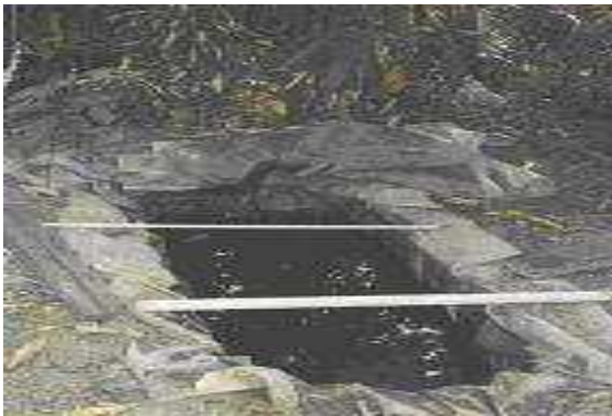
Figure 3a: Above-the-surface tank (Idamelanda) under construction (Credit: Janaki Chandimala)
