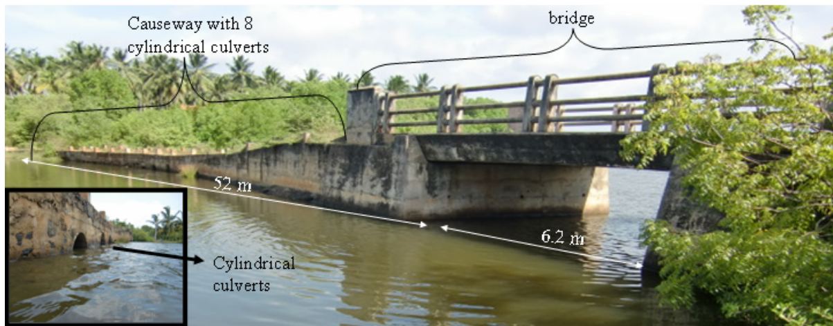
Fig. 2: Existing situation of the causeway with 8 cylindrical culverts and the partial bridge at Kapuhenwala, Rekawa Lagoon
