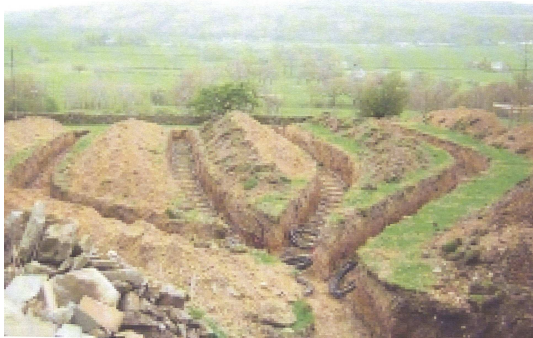
Fig. 6: Shallow horizontal "slinky" ground loops in trenches (Banks, 2008).
