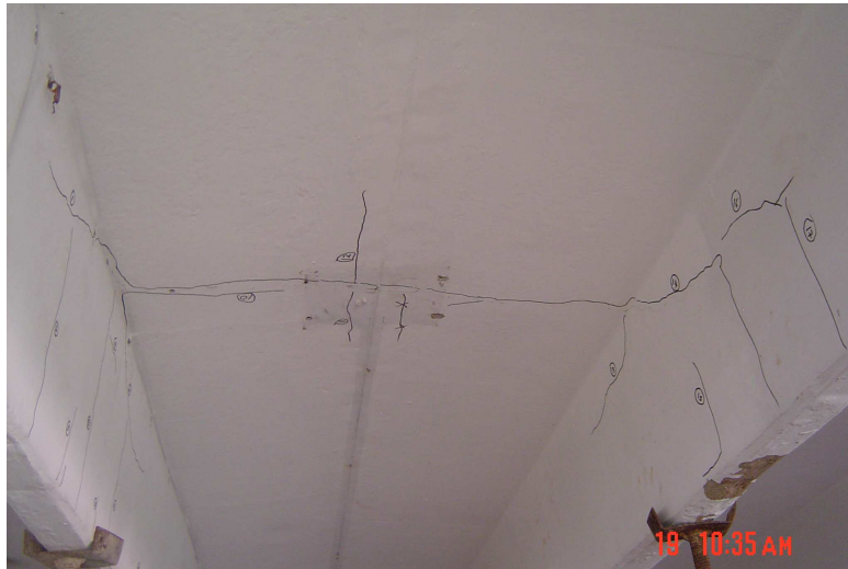
Figure 10: Cracks at T-beams flanges
