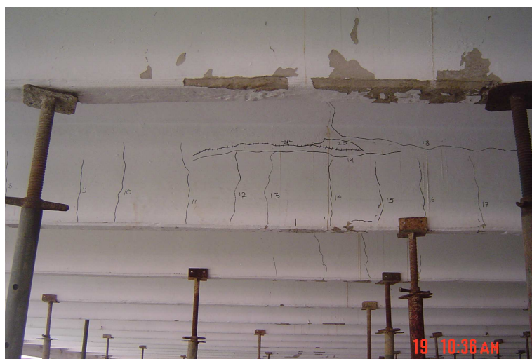
Figure 9: Hair line cracks on T-beams close to mid spans
