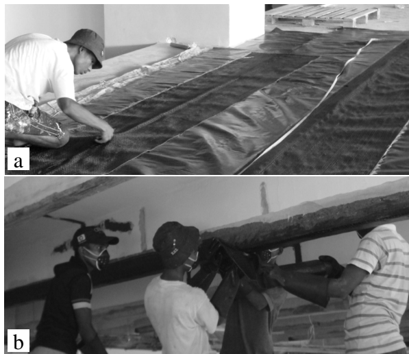
Figure 5. A) sizing carbon fibre fabric. B) instaling saturated fabric onto element.
