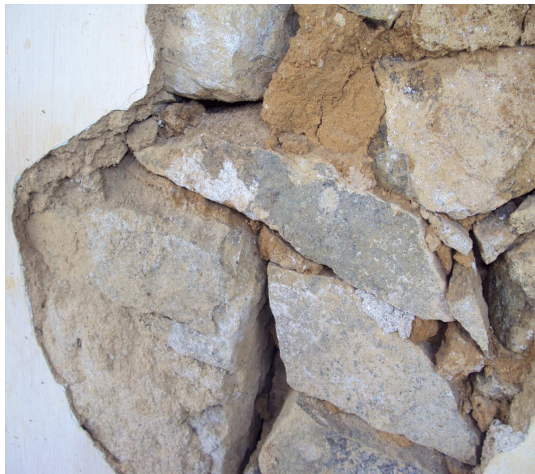
Fig 3.3 Rubble and clay mortar used to build walls in a bungalow at Hanthana, Kandy
