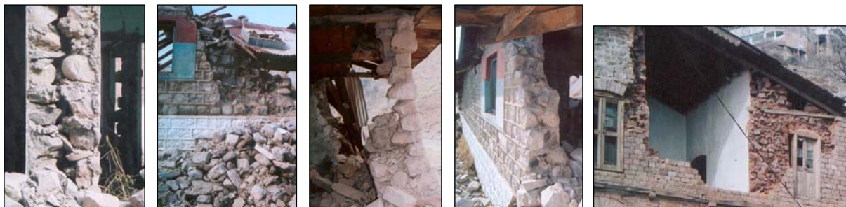
CROSS-SECTIONS OF TRADITIONAL WALL AND COLLAPSED STRUCTURES SHOWING LACK OF BONDING BETWEEN FACES, BUT WITH THE USE OF A LARGE AMOUNT OF CEMENT MORTAR AND PLASTER. LACK OF ANCHORAGE OF WALLS.
