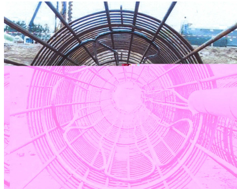
Fig. 9: HDPE ground loops in reinforcing cage of a large diameter pile before vertical installation (Enercret, 2009).
