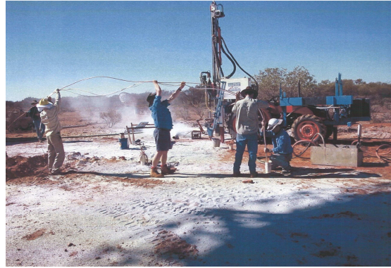
Fig. 5: Installation of copper ground loop into small diameter borehole (Payne, 2010).
