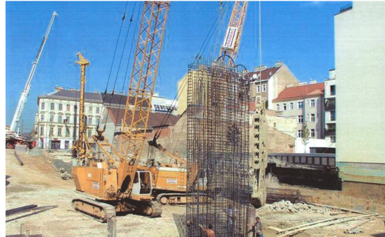
Fig. 7: Lowering HDPE ground loops into the ground on the reinforcing cage of a section of diaphragm wall (Enercret, 2009).
