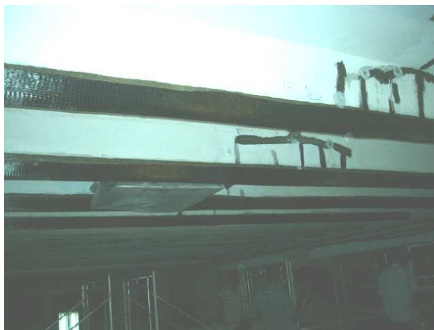
Figure 12: The beams completed with FRP work
