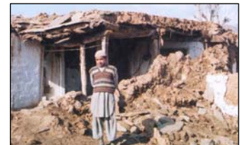
TRADITIONAL HOUSE ~ COLUMNS JUST MANAGE TO KEEP THE HEAVY ROOF UP. WITHOUT THE REMAINING BRACING WALLS, THE STRUCTURE WILL COLLAPSE FURTHER.
