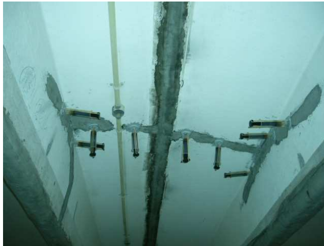
Figure 11: Repairs to non-structural cracks
