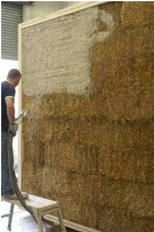
Figure 3. Spraying lime render on ModCell panel
