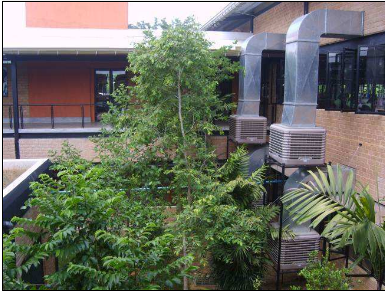
Figure 4: An evaporative coolers installed in a factory building
