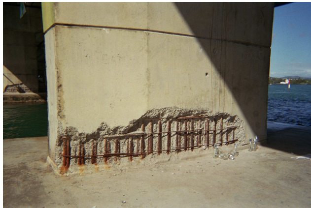
Figure 9 – Damaged Concrete
