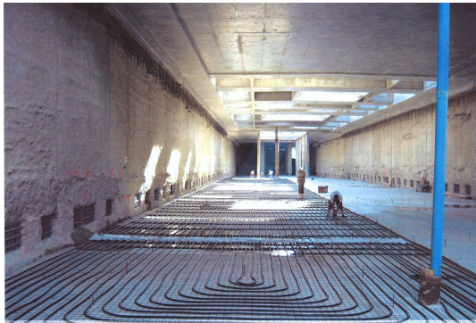
Fig. 8: Horizontal ground loops in a mass concrete base slab (Enercret, 2009).
