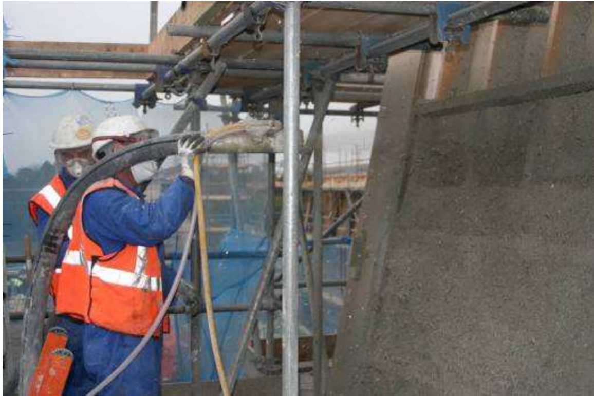
Figure 2. Spraying hemp-lime (Lime Technology Ltd)
