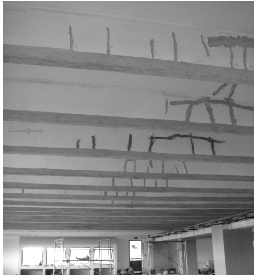
Figure 2. : View of beams showing typical flexural crack patterns.
