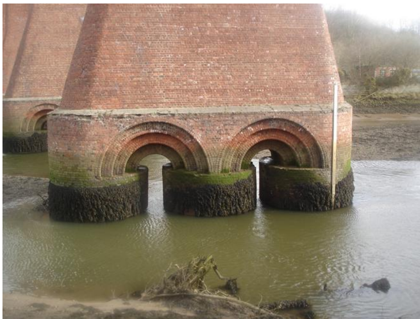
Figure 4. Solid brickwork piers of Larpool viaduct.
