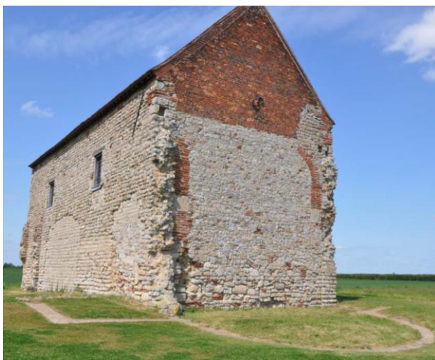
Figure 1. The chapel showing an exposed original clay brick column and the remains of an arch (the roof and gable walls are not original construction).
