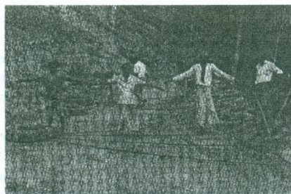
(a) Placement of Anchor Tyres and Facing tyres
