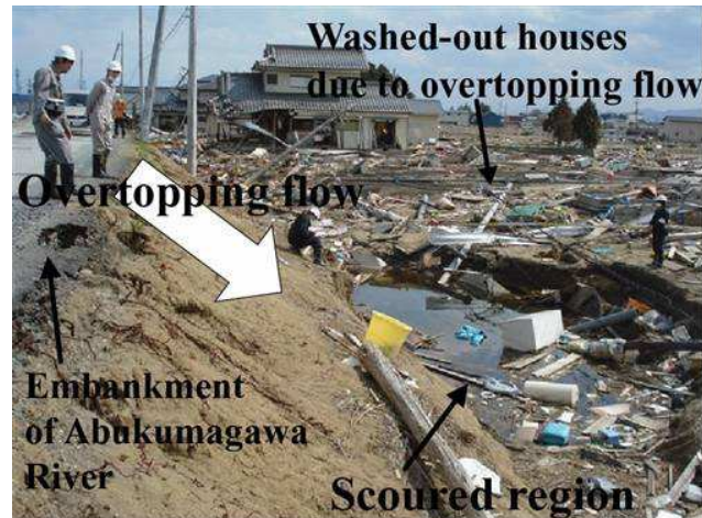
Figure 3 Large scoured region by overtopping flow (Right hand side of Abukumagawa River)
