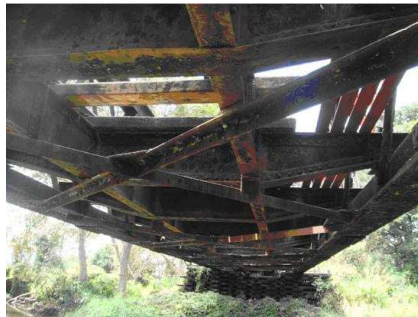
Corroded load carrying elements
