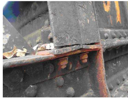
Defective connections
