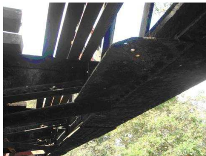
Missing elements and rivets
